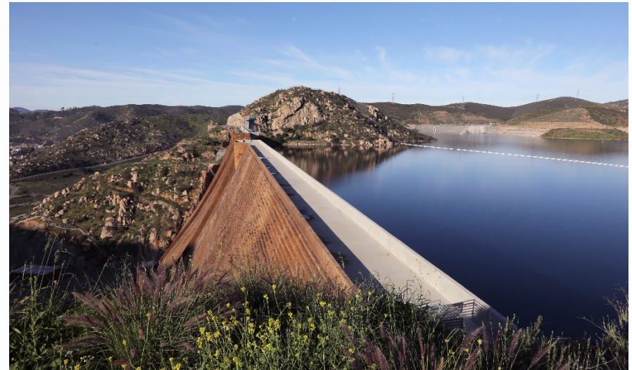
San Vicente Dam
